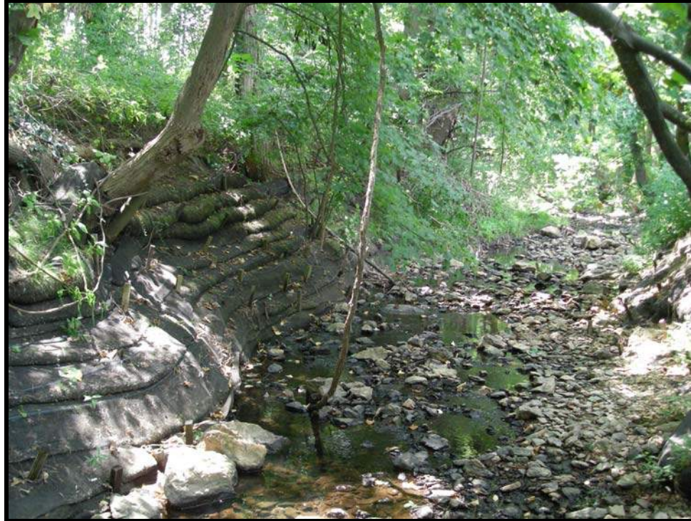
Figure 5: Filtrex Socks at Daniels Run
