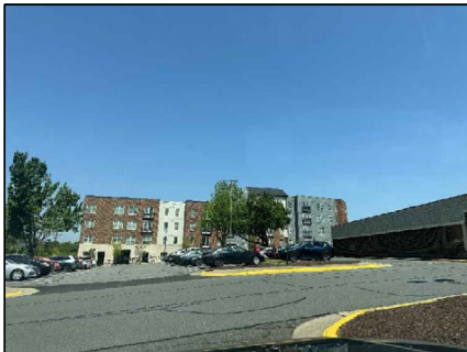
H VIEW LOOKING NORTH FROM INTERSECTION OF PARKING LOT AND UNIVERSITY DRIVE SITE ENTRANCE
