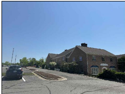
G VIEW LOOKING SOUTHEAST ALONG SOUTHERN DRIVE ISLE FROM SOUTHWEST CORNER OF PARKING LOT
