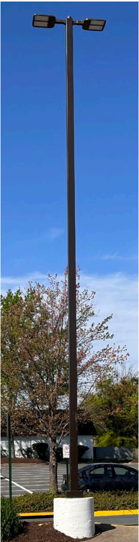
EXISTING PARKING LOT LIGHT FIXTURES CREE LIGHTING - OSQ SERIES
