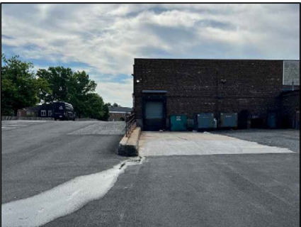
J VIEW LOOKING EAST AT SAFEWAY LOADING DOCK
