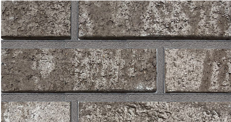
AFB-2 - Brown Brick Brown Mortar
