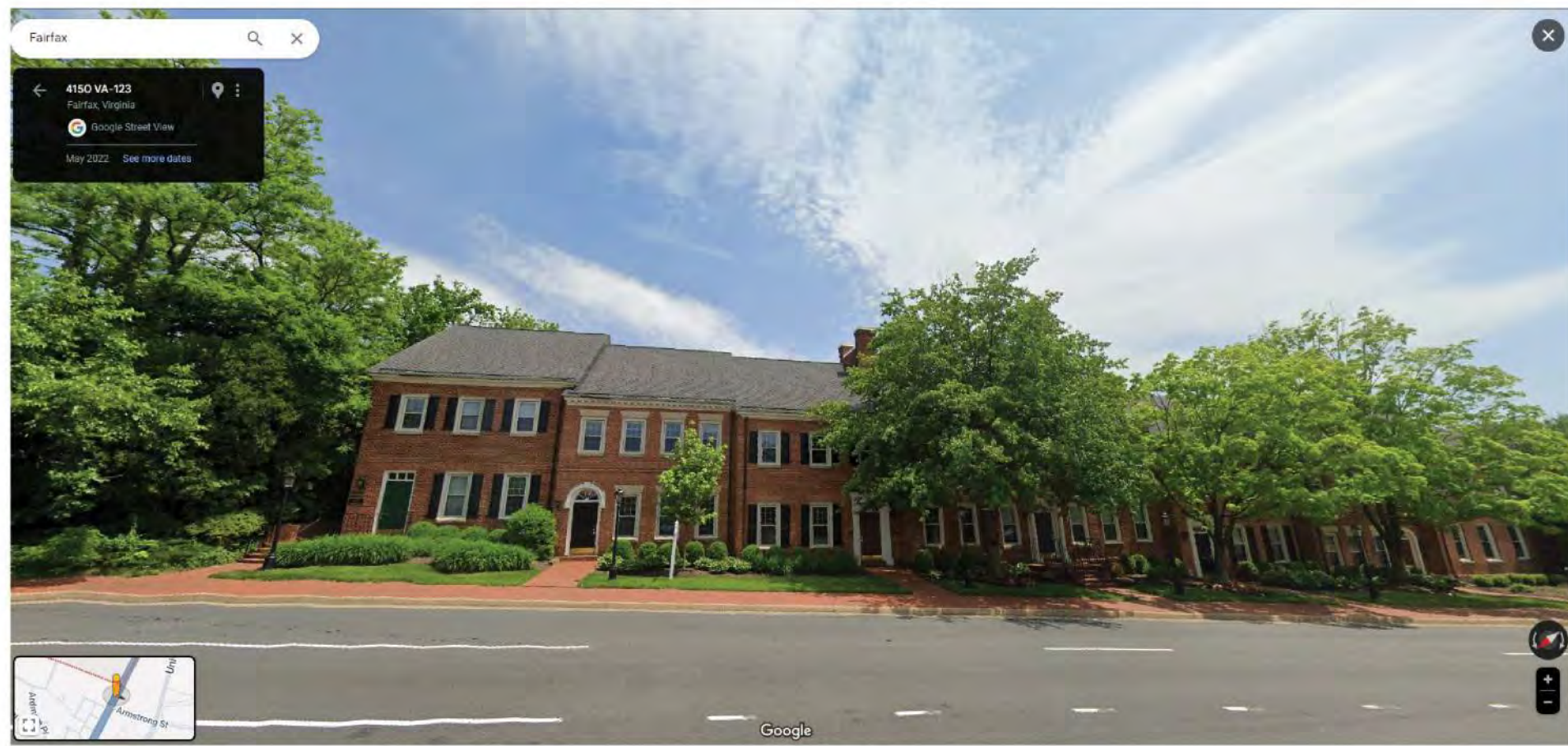
2) CHAINBRIDGE- SOUTH PROPERTY- 1
