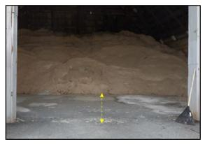
Figure 1. Loose rock salt should be placed deep enough into storage bins to prevent contact with precipitation.
