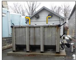
Figure 1. The brine feeder hopper wings must be fully opened (arrows) prior to feeding rock salt.
