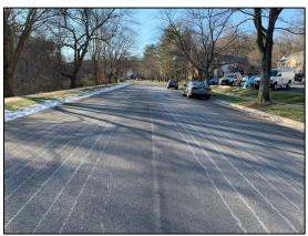
Figure 2. Brine application should result in a repeating pattern of brine and clean pavement with minimal brine runoff.
