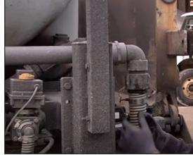
Figure 1. Tightly attach feed lines between the pump house and brine trucks.
