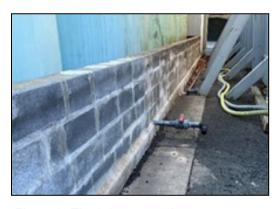
Figure 2. The brine secondary containment drain valve must remain closed when brine is being stored.
