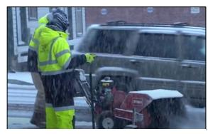
Figure 1. Physically remove as much snow and ice from the infrastructure as possible prior to treatment with chlorides.
