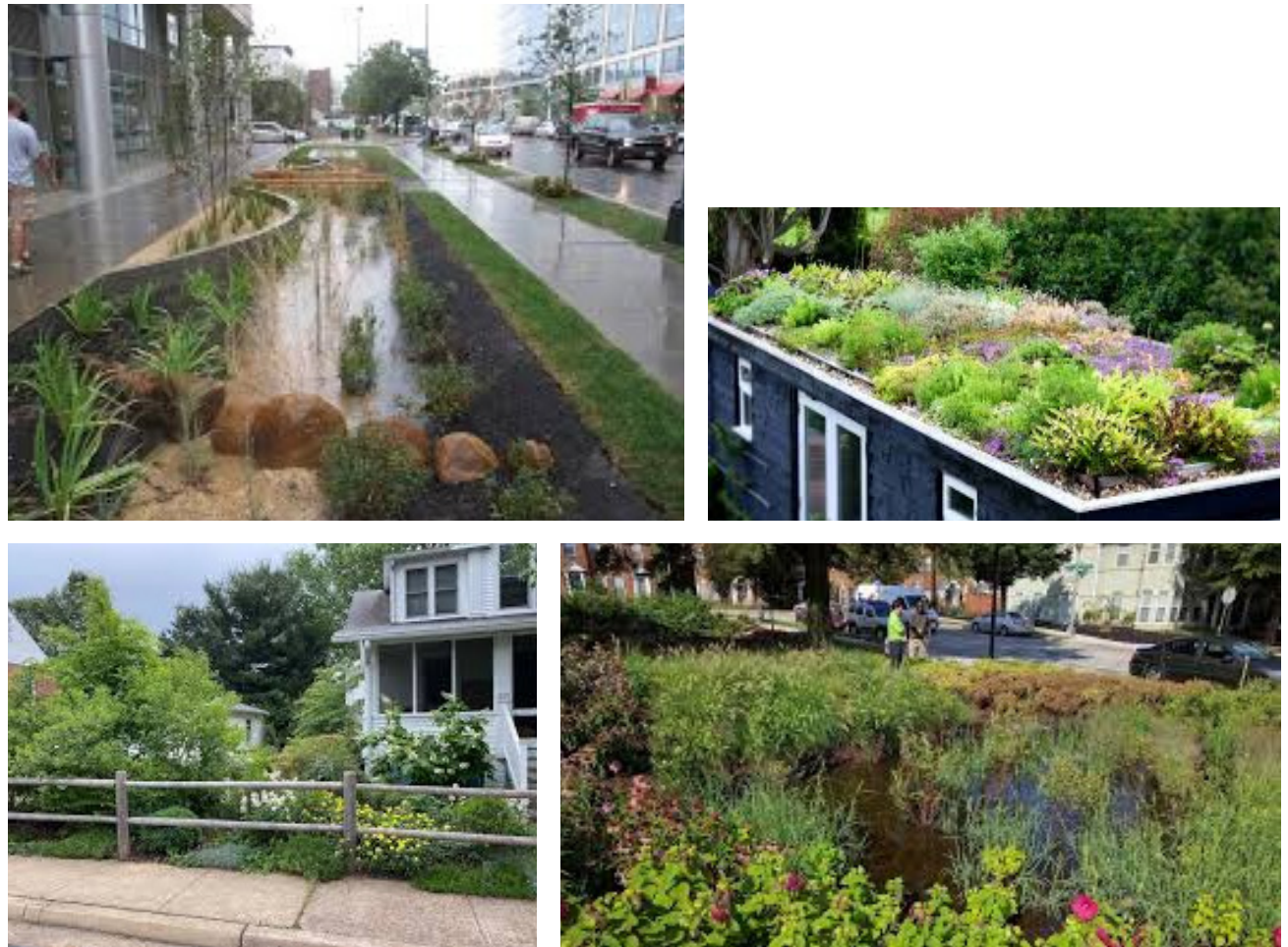
Top Left: Example of a bioswale which collects rain water during storm events and allows it to infiltrate into the soil rather than running to a stream. Top Right: Example of a green roof which reduces run off and can be used to harvest stormwater. Bottom Left: Sustainable landscaping with plants native to Northern Virginia and habitat for pollinators. Bottom Right: A rain garden populated with native plants that can provide a habitat for native species and help with stormwater management.
