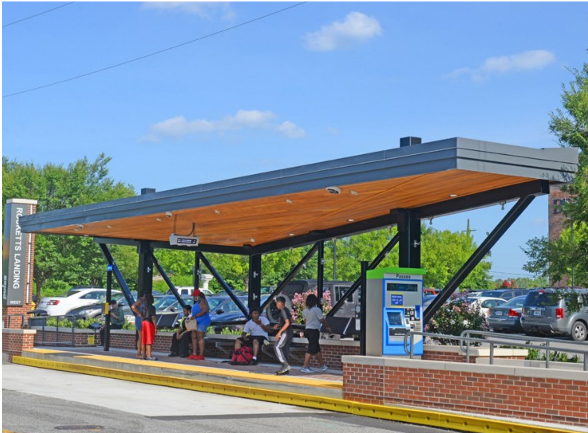
Example- Transit Shelter - Richmond, VA
