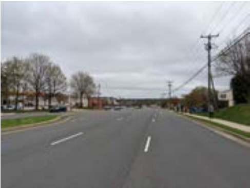
NARROW SIDEWALKS NEXT TO WIDE ROADS
