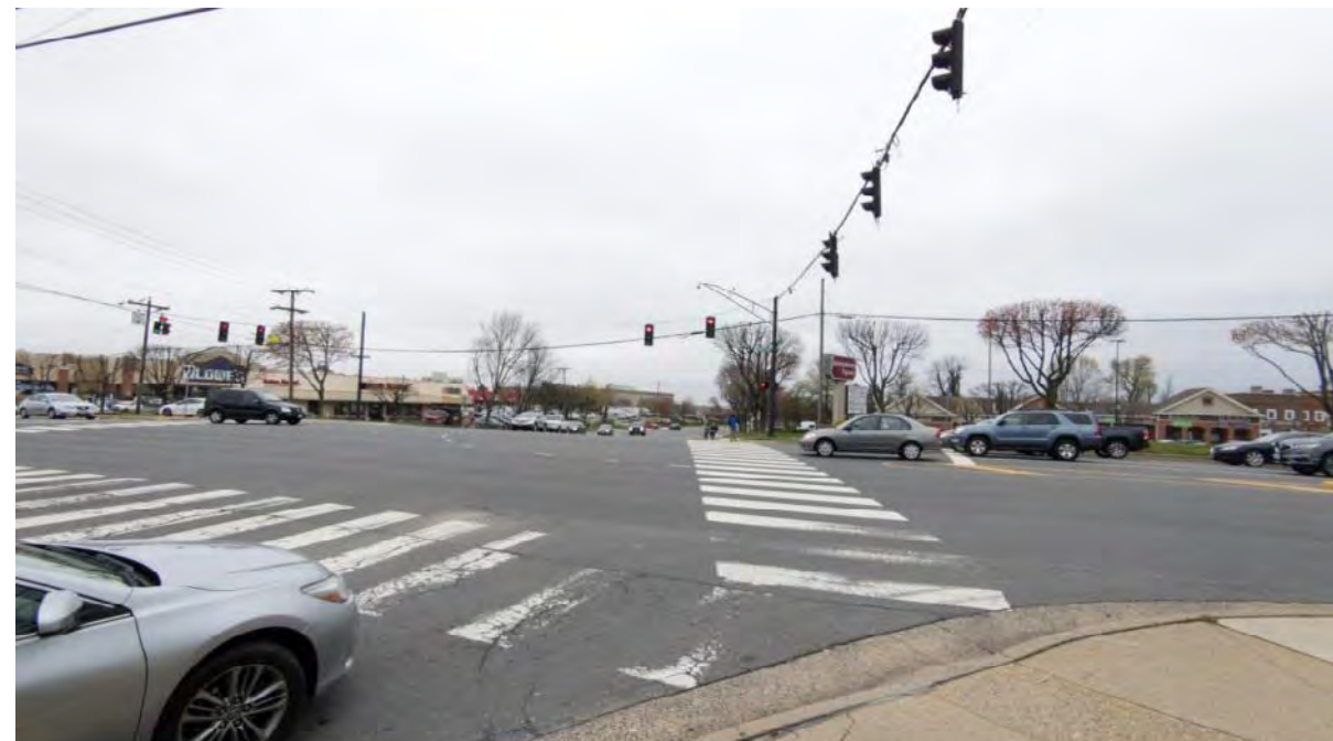
Narrow corners with non-ADA compliant ramps and Long crosswalks without any refugee islands
