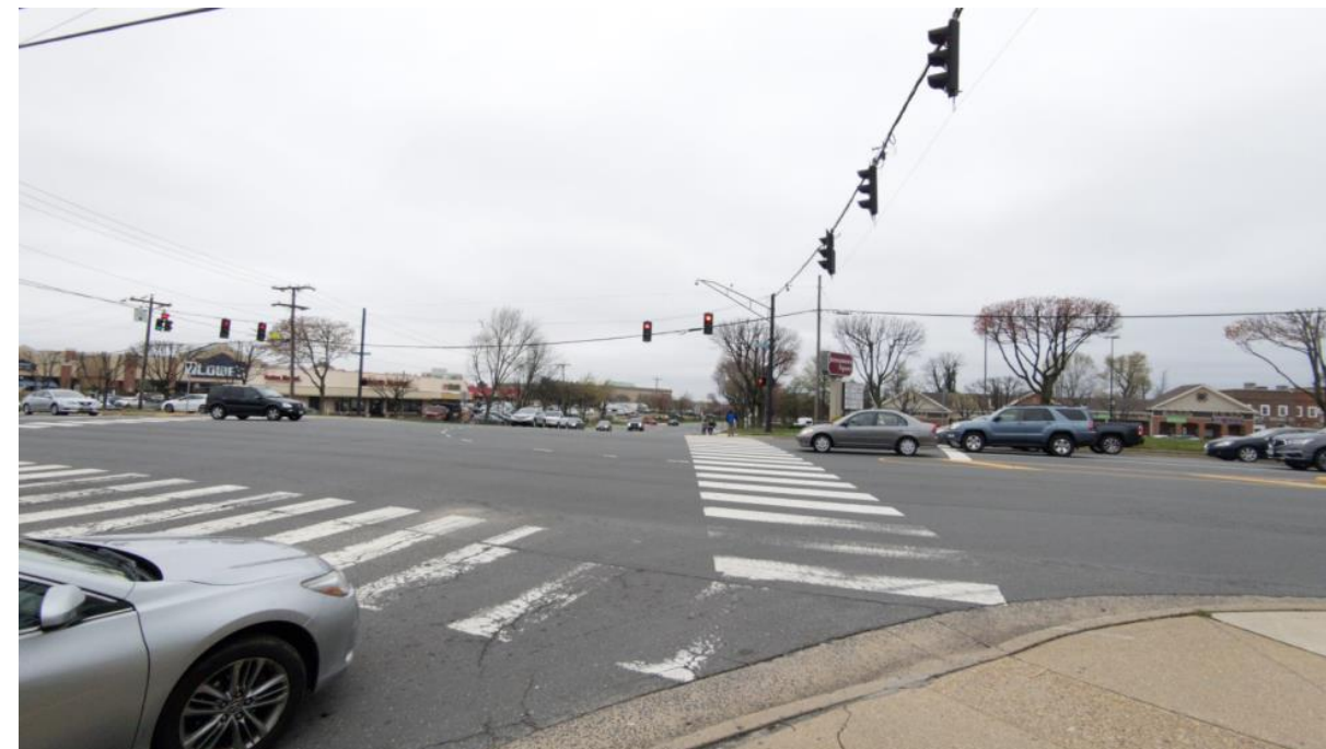
Narrow corners with non-ADA compliant ramps and Long crosswalks without any refugee islands
