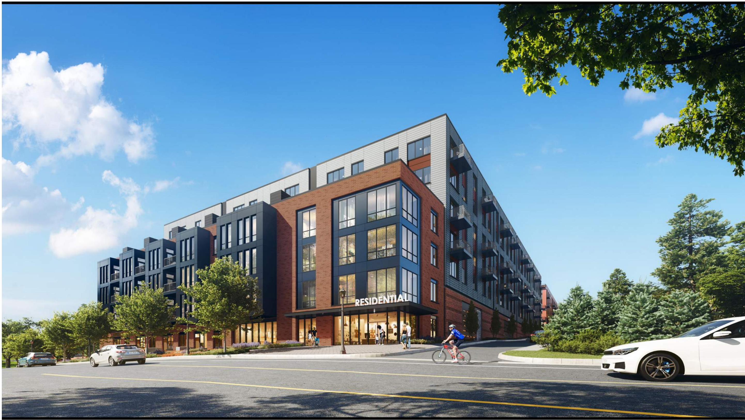
① UNIVERSITY DR VIEW LOOKING SOUTHWEST
