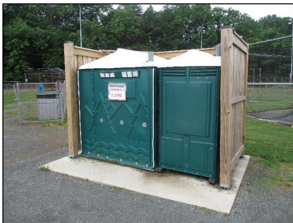
Figure 12. Park portable sanitation facility with protective barrier (2020)
