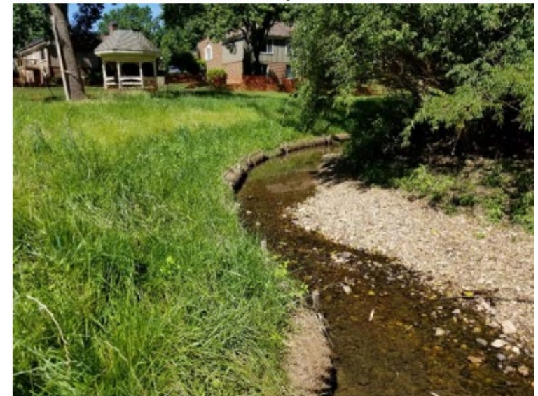
After Construction & Stabilization, June 2020
