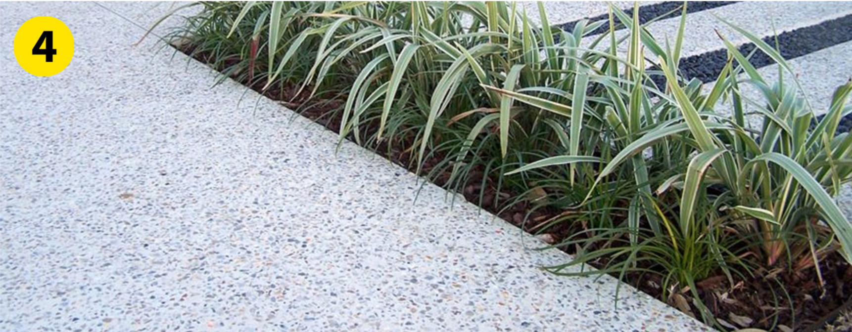
EXPOSED AGGREGATE CONCRETE PATHWAY AT CEDAR AVENUE
