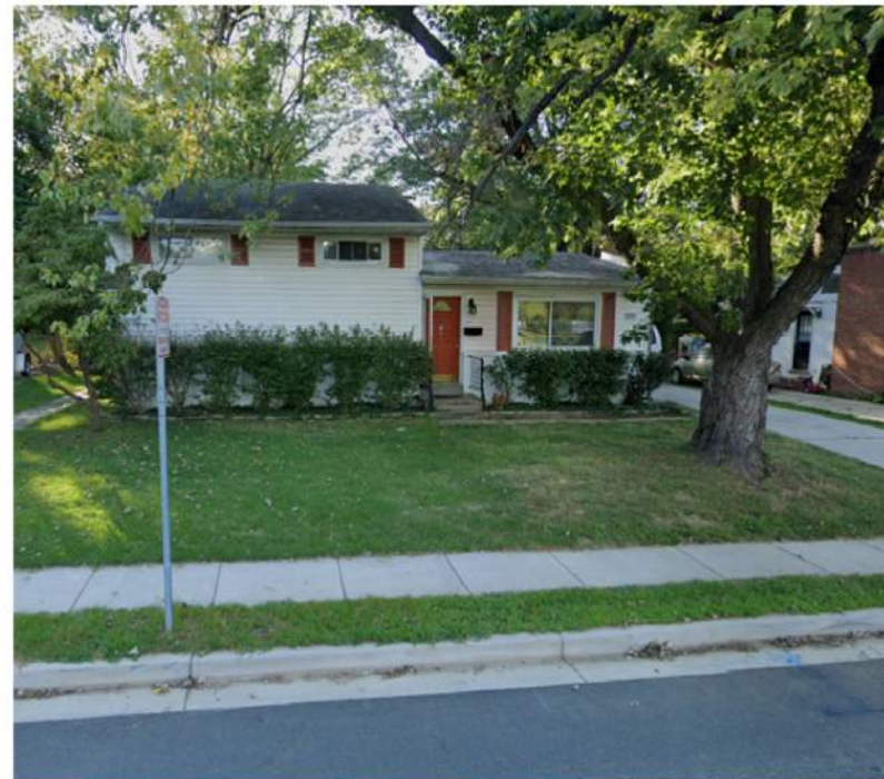
Single Family Home along Oak Street
