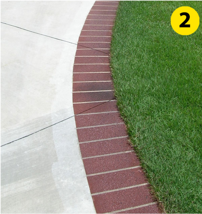
BRICK EDGING AT CONCRETE
