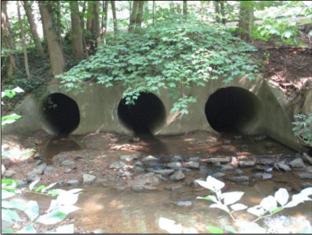
Figure 10. Triple 60" Culvert Inflow
