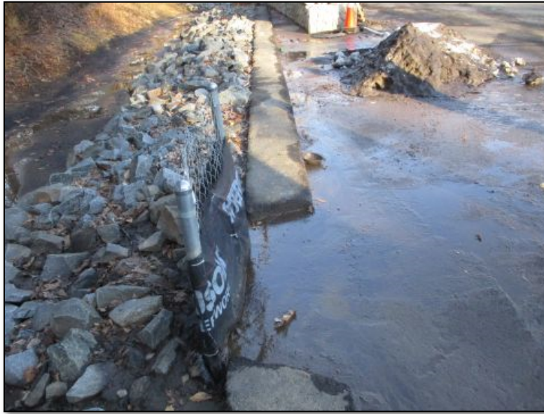
Figure 5. Curb and Silt Fence Installation (2020)
