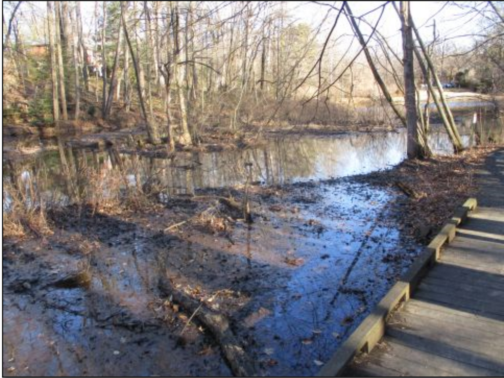
Figure 7. Ashby Pond Sedimentation and Existing Forebay Area
