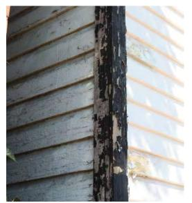
Paint failure can occur when wood is not properly primed.
