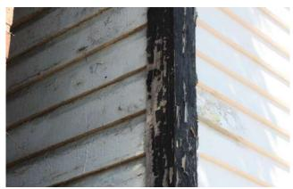
Wood must be maintained by regular painting to prevent deterioration.
