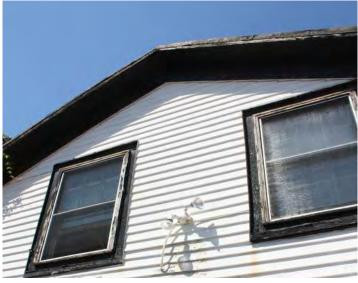
A inspection of the subject building reveals condition issues like this paint failure and may also require further investigations to determine if sections of the wood trim need to be replaced as well.
