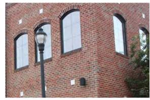
While this window shape and masonry detail of this new building reflect traditional openings, the windows appear more like a single sheet of glass and muntins are barely visible.
