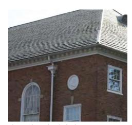
This conductor head, also known as a scupper, helps to drain this hidden gutter.
