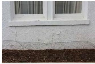
Stucco surfaces are susceptible to water infiltration.
