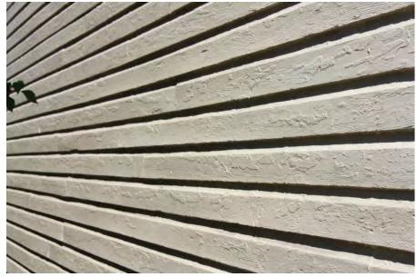
Historic wood siding may have multiple layers of paint after many years of repainting. At some point, the paint build-up begins to fail (known as alligatoring) and additional layers will not adhere. At that point, the old layers need to be removed down to the original wood and the siding prepped, primed and repainted.
