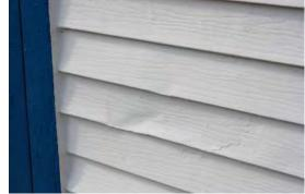
Artificial siding can be dented and in these cases, is difficult to match material and replace the damaged piece.
