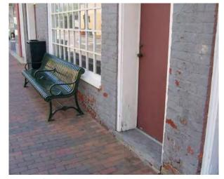
Moisture from below grade (known as raising damp) can cause paint failure on masonry.
