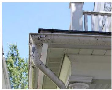
Without proper cleaning and the recommended primer, paint failure may occur on galvanized gutters and downspouts.
