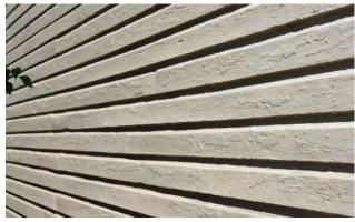
Excessive paint layers eventually will result in the failure of paint to adhere.
