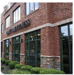
The brick facade on this example is supported by stone bases on the piers.
