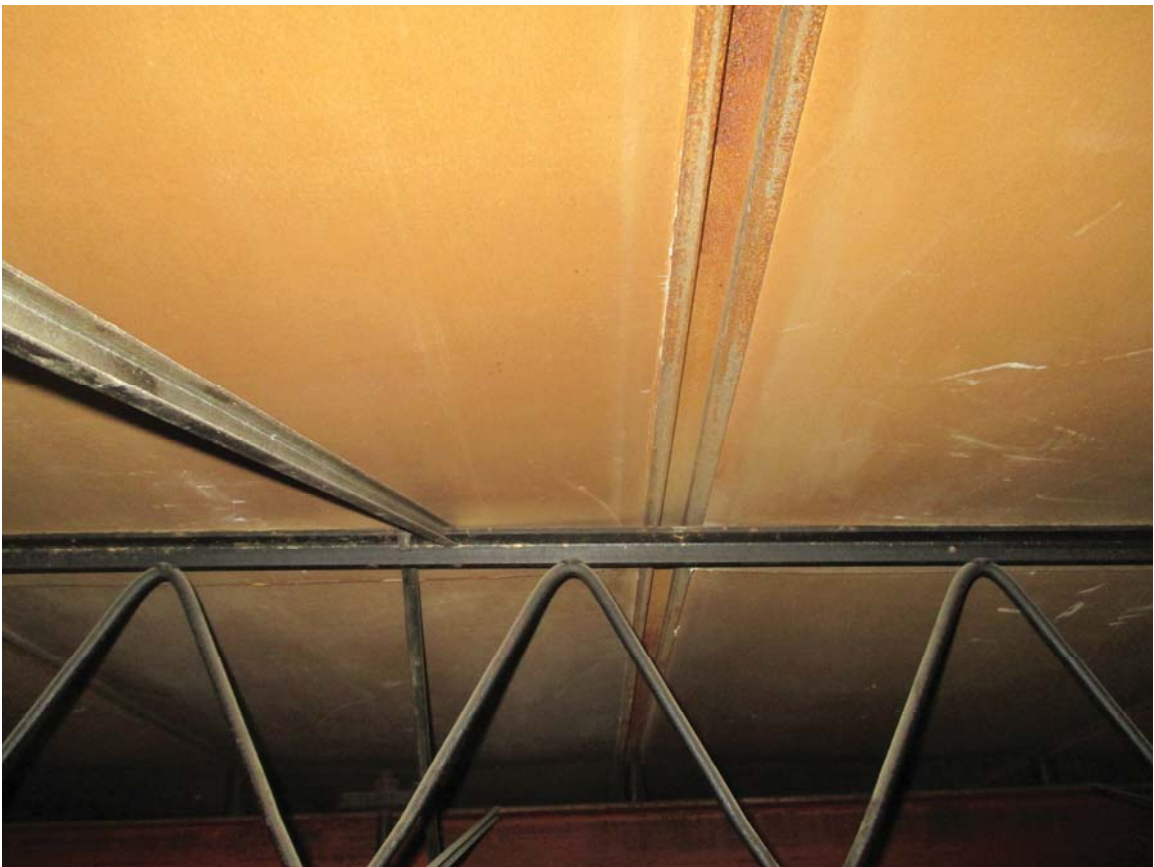
Photo #3: Roof deck spanning across an open web steel joist
