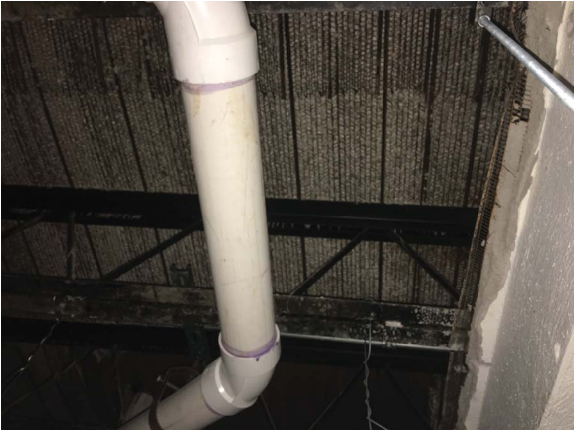
Photo #2: Open web steel floor joist with draped mesh supporting a concrete floor slab.
