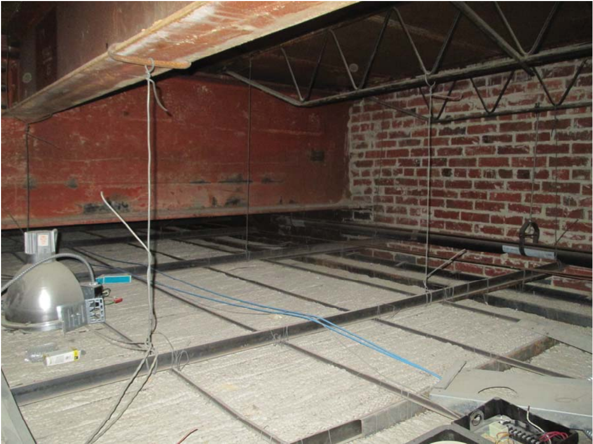
Photo #4: W36 roof girder bearing into adjacent masonry wall
