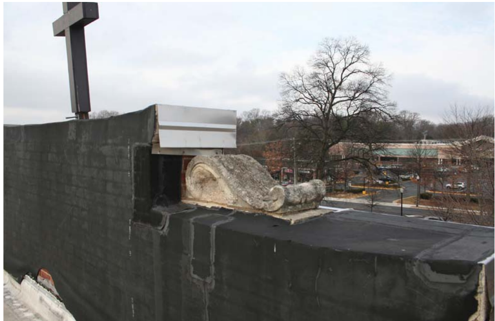
Back of Parapet with hole and deteriorated cast stone
