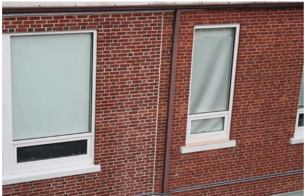
Rear Wall West Courtyard, original brick wall on right side of expansion joint
